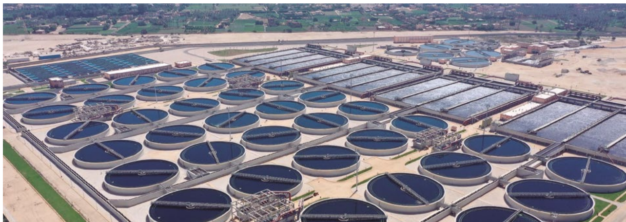
Abu Rawash wastewater treatment plant, Egypt.
